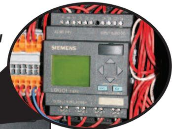
**Smart Relay Control** provides complete control over run time, auto start/stop and time delay shut down functionality.
