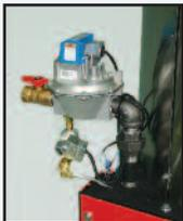
**Burner assembly** pivots down to allow access to burner ring and pilot assembly for maintenance
